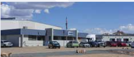
Distribution Center, Kingman, Ariz.
