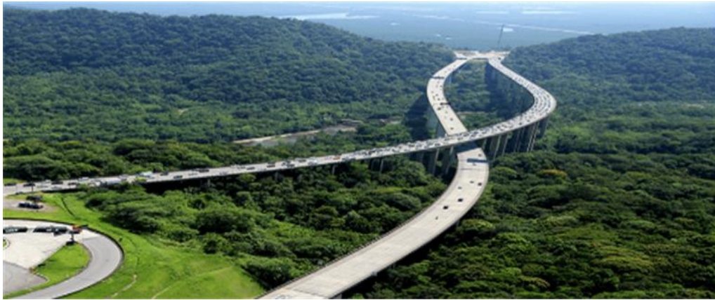
Chart 12 – Example of a bridge entrusted to Argan
