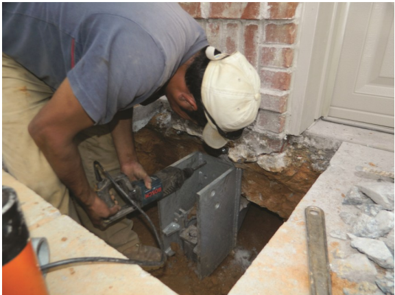
Lift and secure a foundation
