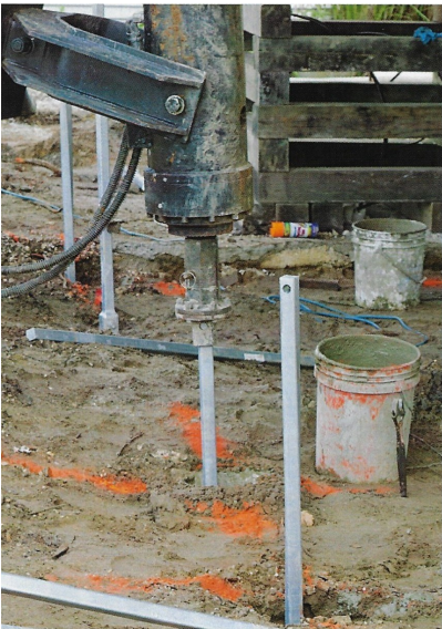
Helical piers for new construction
