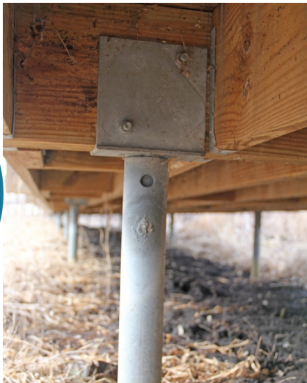
Lift and secure a foundation
