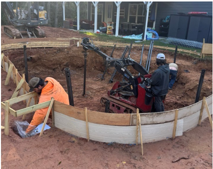
Securing a deck
