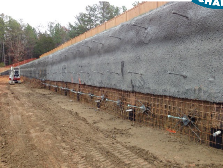
Tie Backs holding a sheer dirt cut
