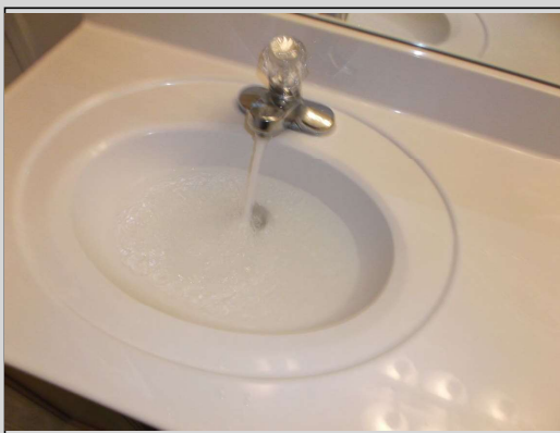
Left sink water slow to drain out
