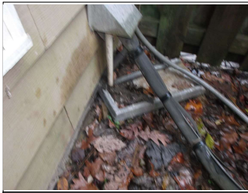
Condensate pipe not extended away
