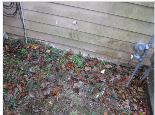
Some of the rear wall installed off the slab
