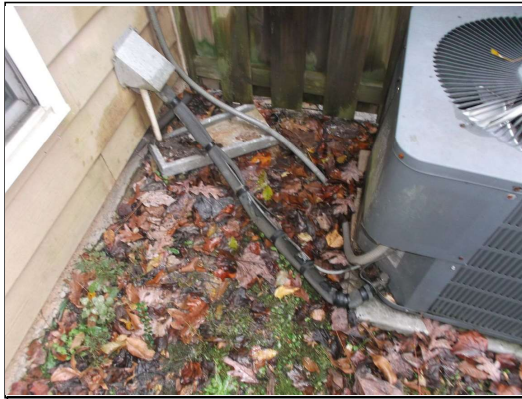
Refrigerant line insulation deteriorated
