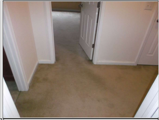
Front bed floor slopes to master doorway
