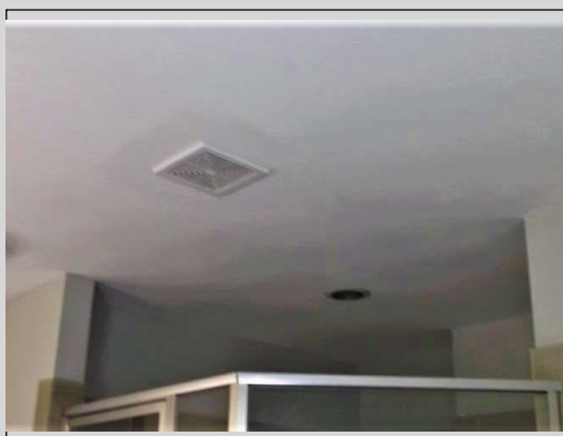
Paint patching in the master bath ceiling
