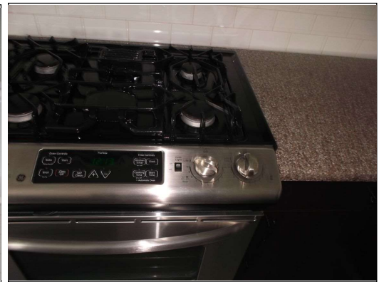
Rear right burner not operational
