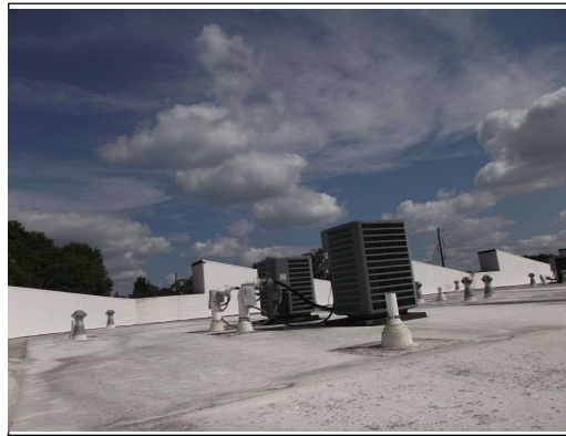
Penetrations in roof near master bath ceiling
