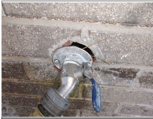
Opening in the brick veneer
