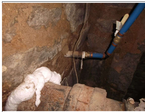
Main pipe in foundation appears to be steel
