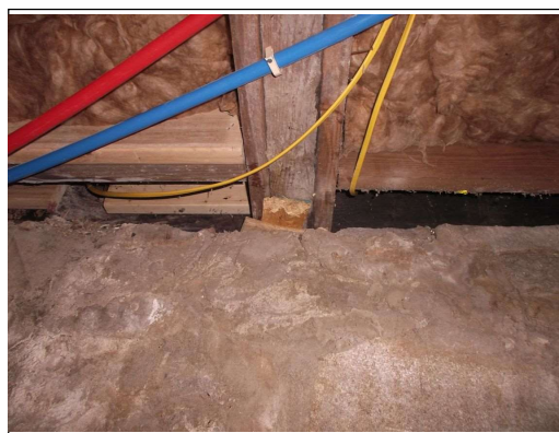
Cannot verify wood is treated on masonry
