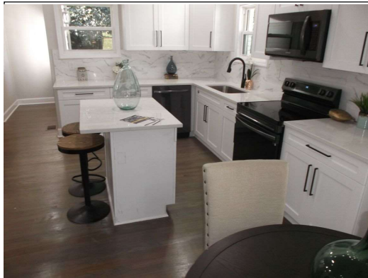
Floor slopes to the sink
