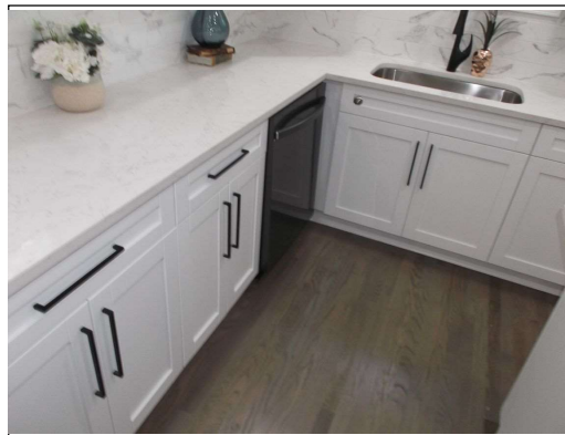
Dishwasher not plumbed
