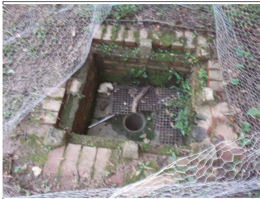
Open pit in rear yard
