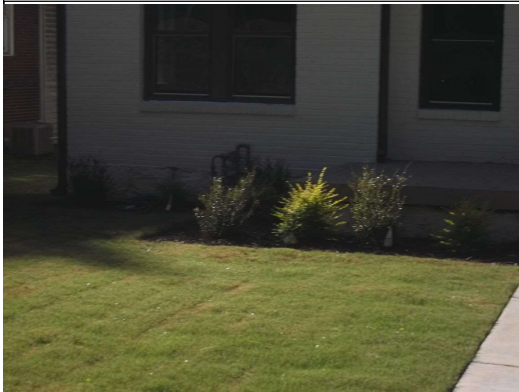
Soil slopes to the front of the house
