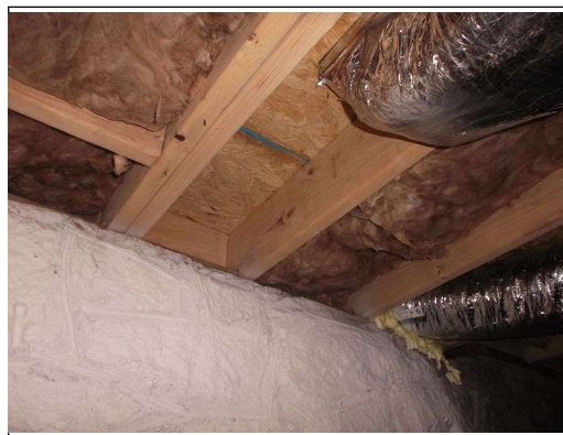
Missing insulation
