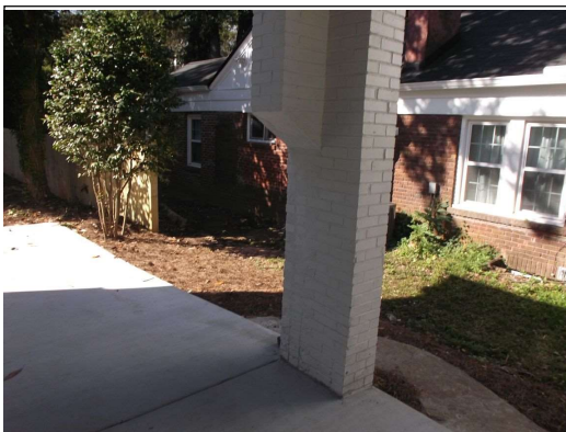
Brick removed at the bottom half of column
