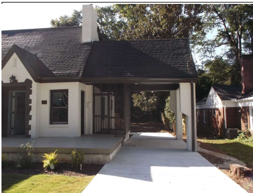
Roof structure slopes to the right
