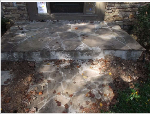
Porch stones repair, high step up
