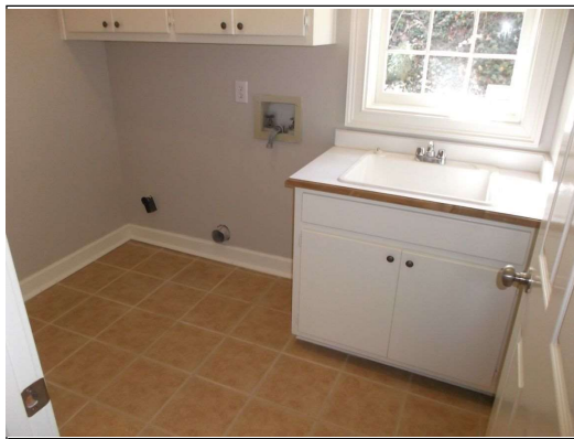
No washer drain pan
