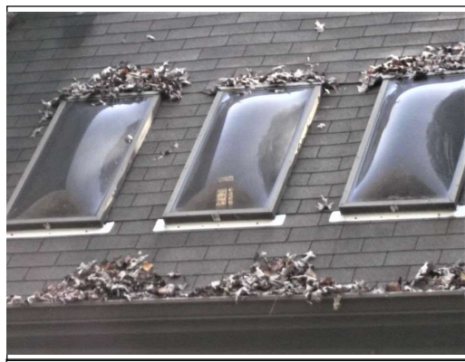
Sky light flashing screws in bottom flange
