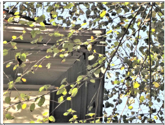
Gutter leaking and water damage to soffit
