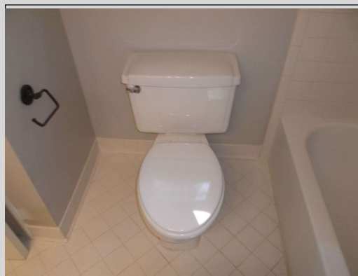
Toilets not water savers
