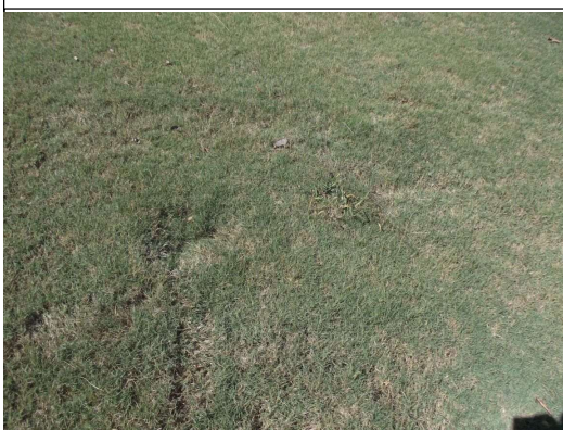
Sink holes in yard
