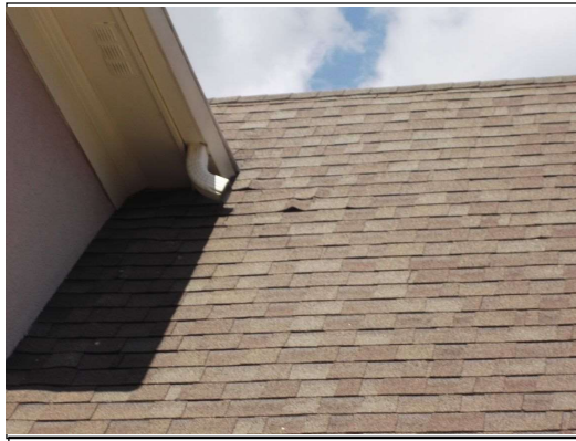
Defective shingles
