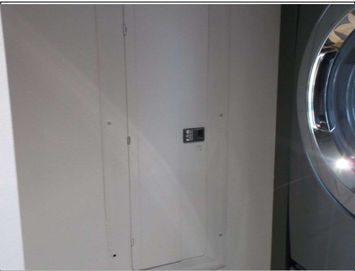
Panel cover sealed to the wall (paint, mud)
