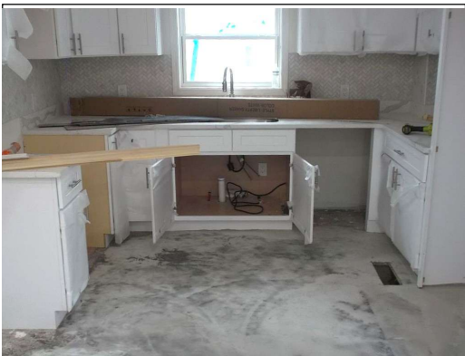
Verify counter not sloping left and right
