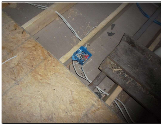
Open junction box in the attic, check all
