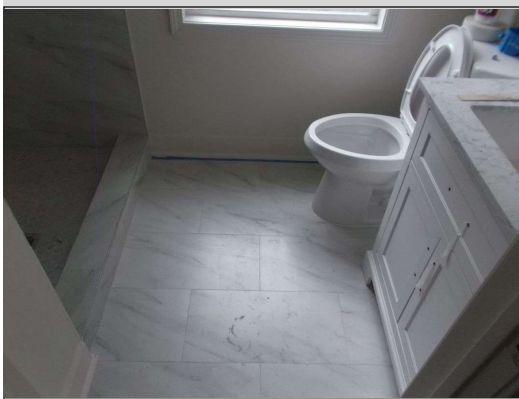
Main bath in final stage of completion
