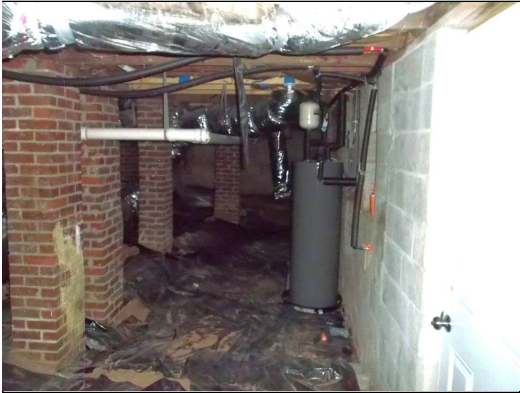
Basement rear area, insulation backwards
