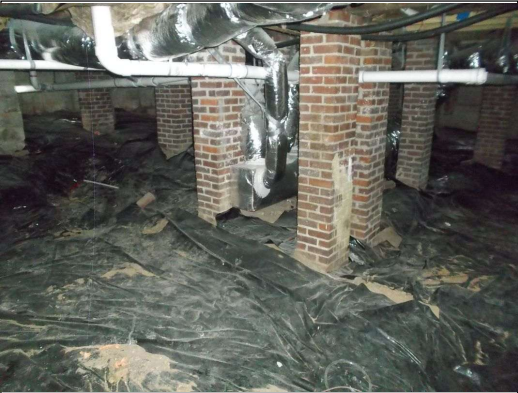
Could not see all areas of the basement
