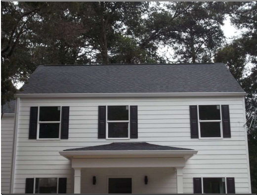
Missing spout right side, porch roof slope left
