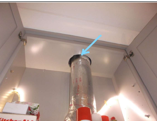
Opening where vent pipe pass through ceiling
