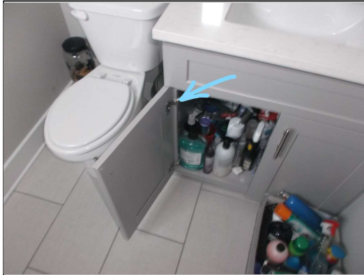
Rear bed bath cabinet door hinges loose
