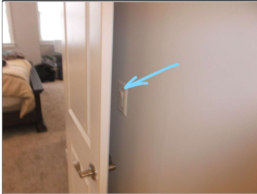
Master bath light switch located behind door
