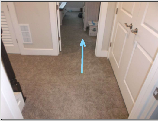
3rd floor hall slopes towards the rear bed
