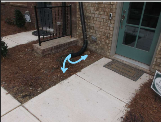
Soil slopes to the front of the building
