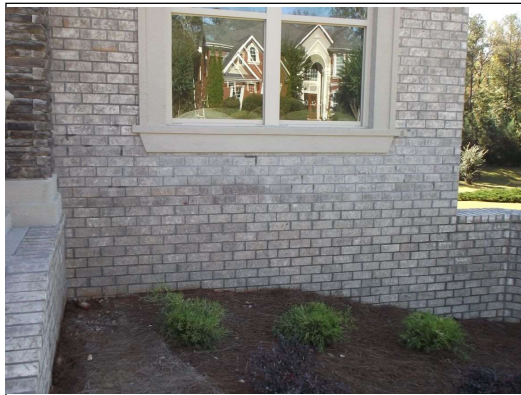
Verify brick color and mortar color
