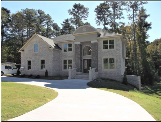
Driveway has excessive slope, dip to the right
