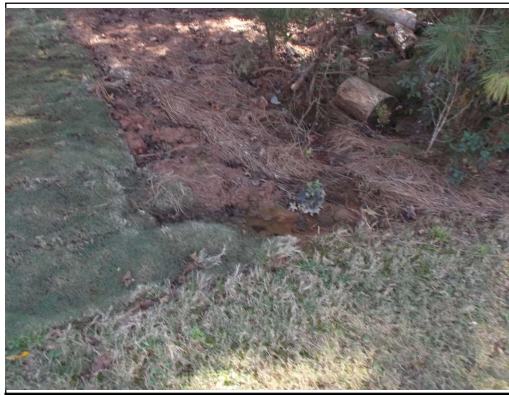
Water in the ground at the rear yard
