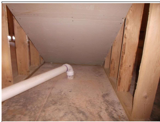
Verify termite shield in place
