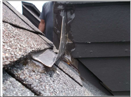
Flashing turned slightly up can drain back
