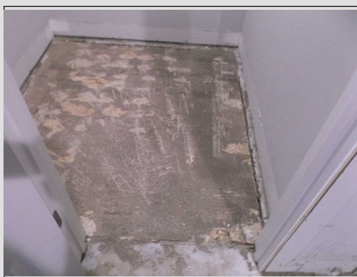
Wood sub floor in concrete floor 1st level
