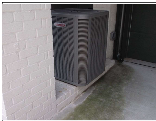
The AC unit is placed in neighbors path
