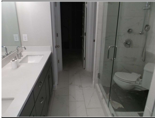
Toilet removed at master bath
