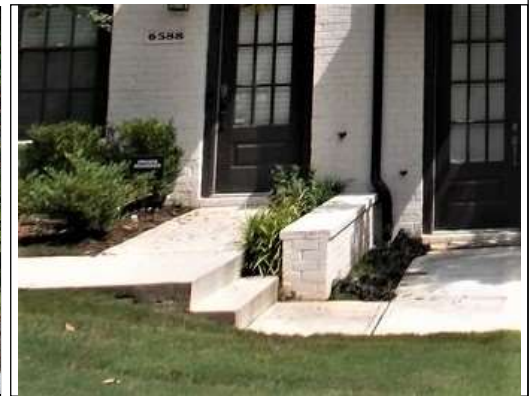
Bottom step blocks drainage from soil
