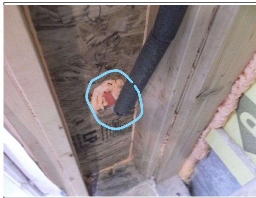
Missing insulation
