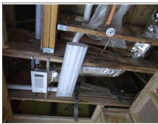
Verify no pipes are leaking
