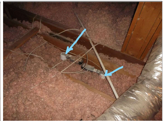
Verify ceiling lights are rated insulate contact
