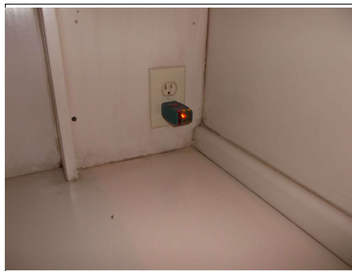
Outlets tested open ground master bed
