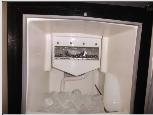
Water kept flowing into the bar icemaker
