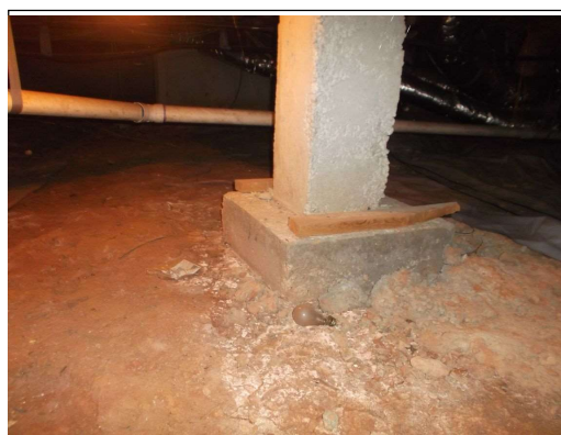
Foundation supports installed on top of soil
