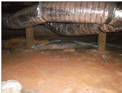
Wood posts alternates placed for masonry
