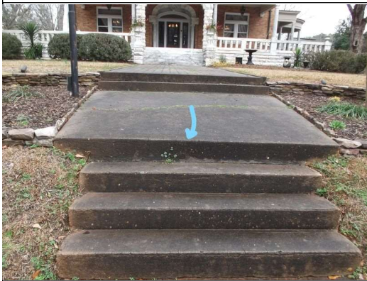
Front main walkway rotates forward at stairs
