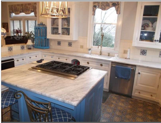
Kitchen outlets not GFCI protected near sink
