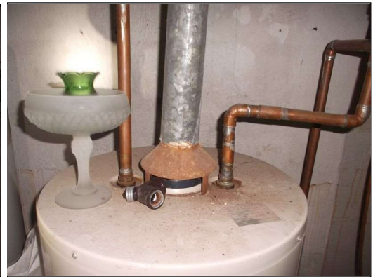
Copper & steel join without dielectric fittings
