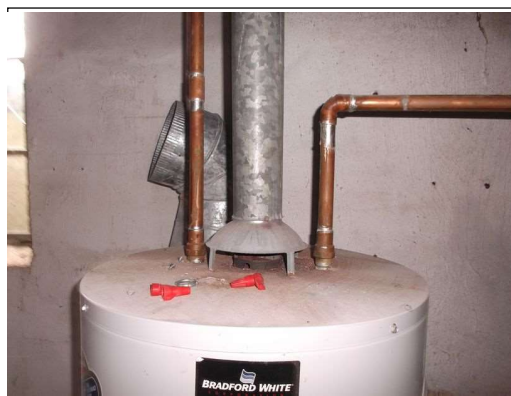
Copper & steel join without dielectric fittings
