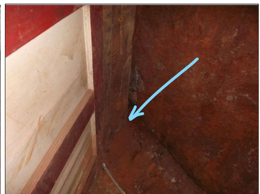
Wood wall framing in the soil
