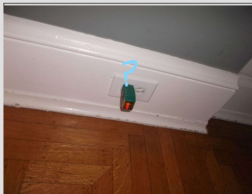
Hot and neutral reversed at bedroom outlet
