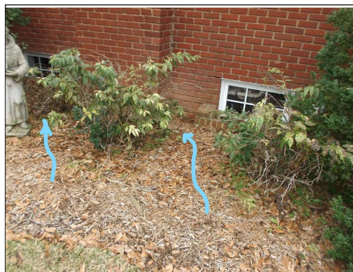
Soil slopes to the building at the right side
