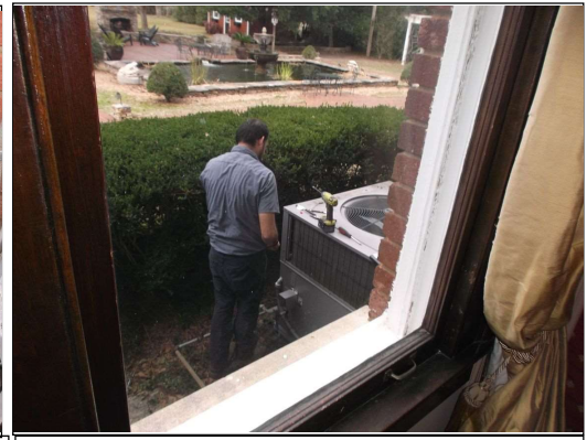
HVAC Tech was working on systems
