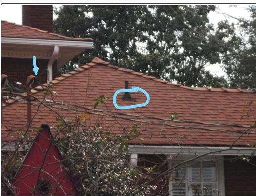
Flashing installed on top shingles face nailed
