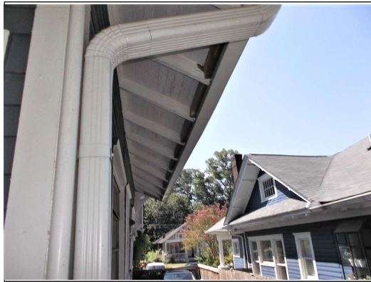
Blocks placed under the roof deck eave
