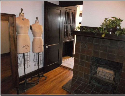
Door drags on threshold, lock loose
