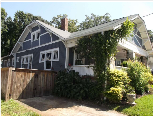
Railings too low, bushes need cut back
