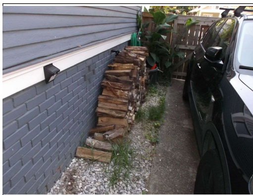
Wood stacked at the foundation
