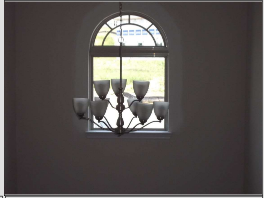
Incomplete finishing and painting
