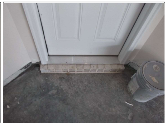
Threshold not supported
