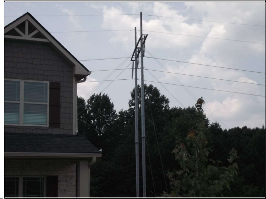
High power utility lines
