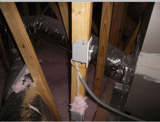
Furnace conduit not clamped to wood
