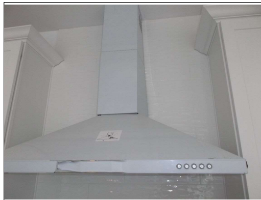
Stove exhaust hood shaft bent right side
