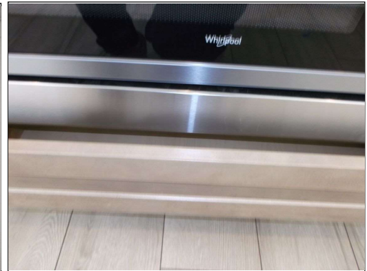
Drawer not closing under microwave
