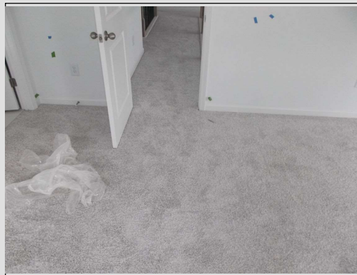
Hump in master bed floor near door
