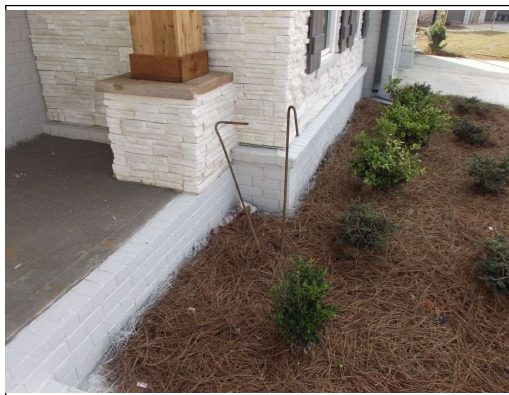
Rebar rising out the ground
