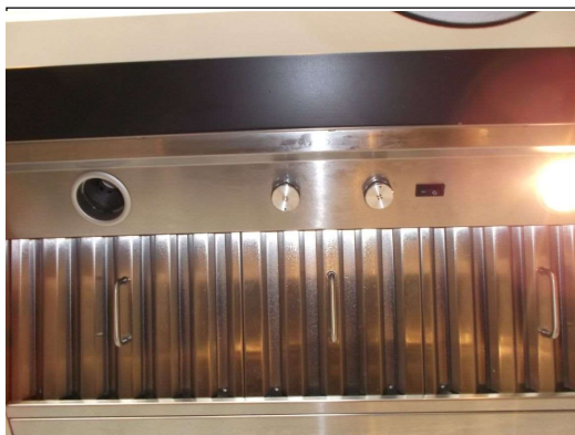
Left light out on the exhaust hood
