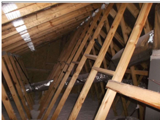
Blocks nailed to the sides of roof truss
