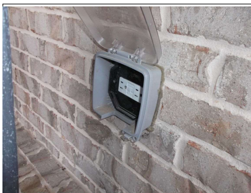
Could not plug into lower front ext. outlet
