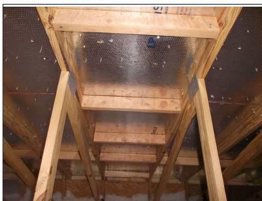
Blocks nailed to the sides of roof truss
