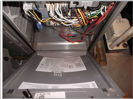
Inside of basement furnace
