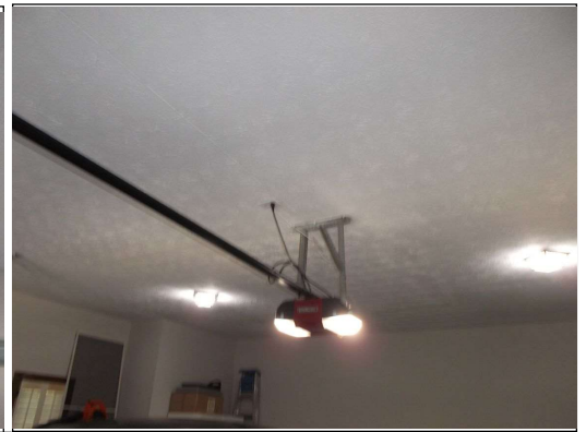
Can see tape seam repairs
