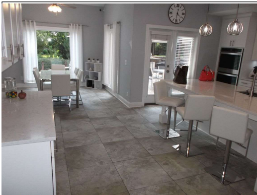
Floor slopes to rear exterior wall
