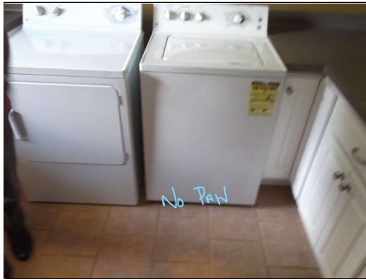
No washer drain pan
