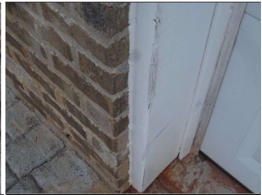
damage to vehicle door frame
