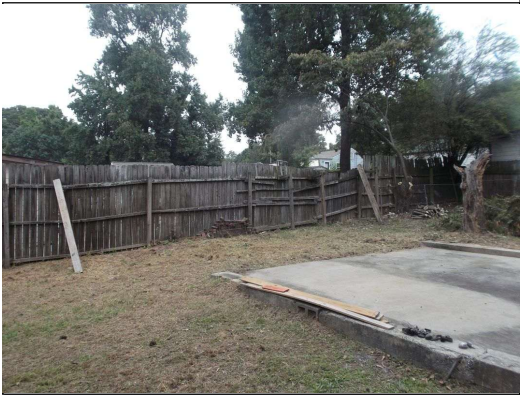
Wood fence damage at areas
