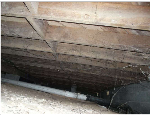
ABS black plastic waste pipe at foundation
