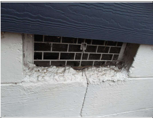
Vents damaged
