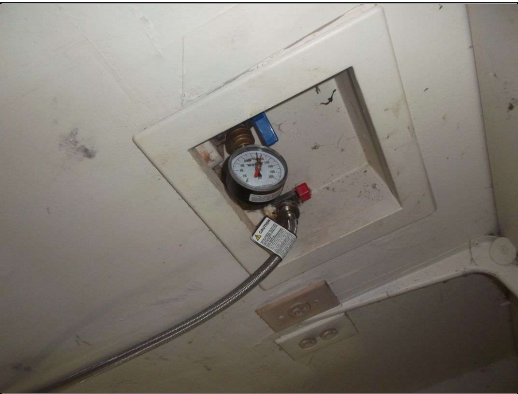
Water pressure over 80 psi
