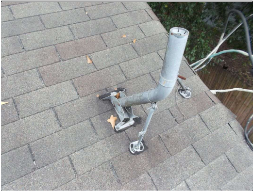
Dish pole bolted to the roof
