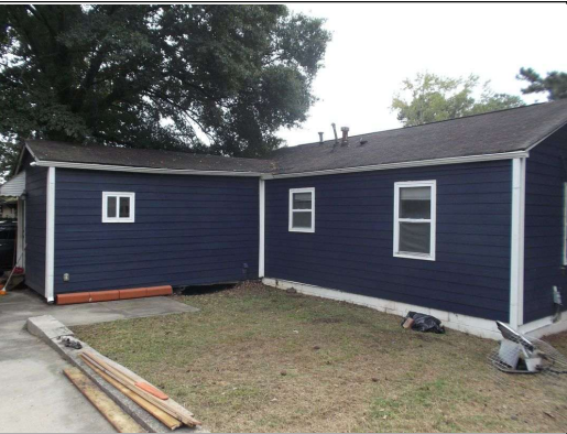
Soil slope to the foundation
