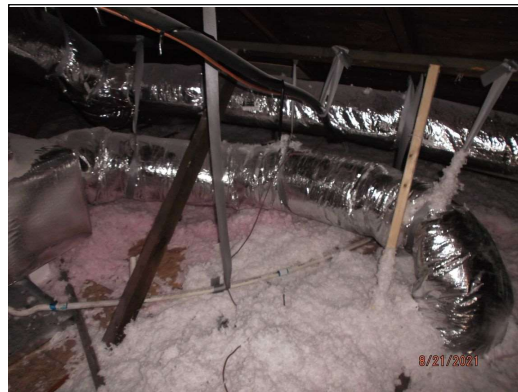
Single 2 by 4s for braces should be two
