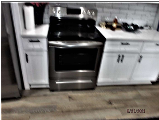
No anti tilt device connected to stove
