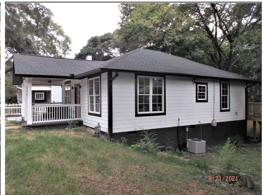
Window screens missing
