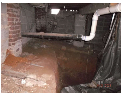
Original cast iron waste pipe
