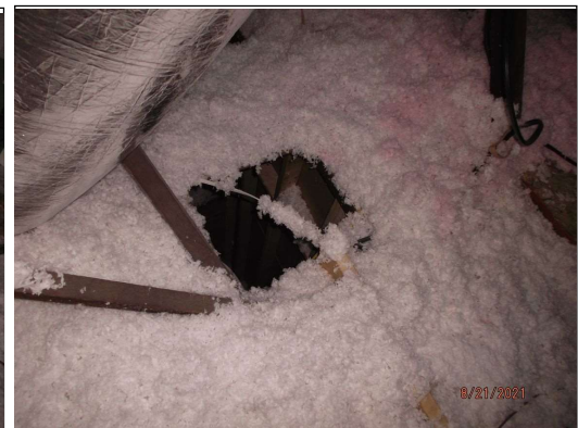
Open chase in attic floor
