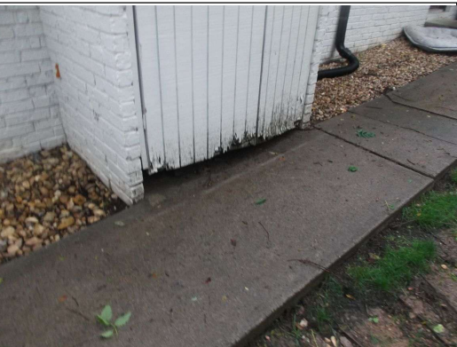
Doors rotted at the 1st meter room
