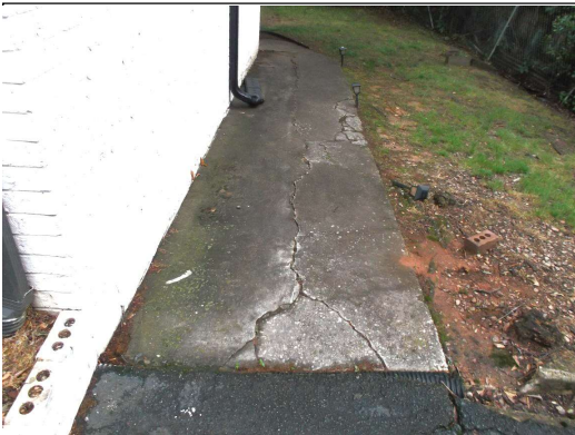
Walkway at right side cracks, broken, slope
