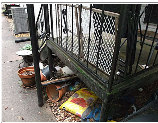
Rail posts at #13 rusted through and loose
