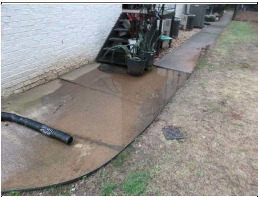
Walkway behind 15 settling, trip hazard, water
