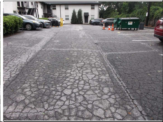
Parking lot has moderate cracking, wear...
