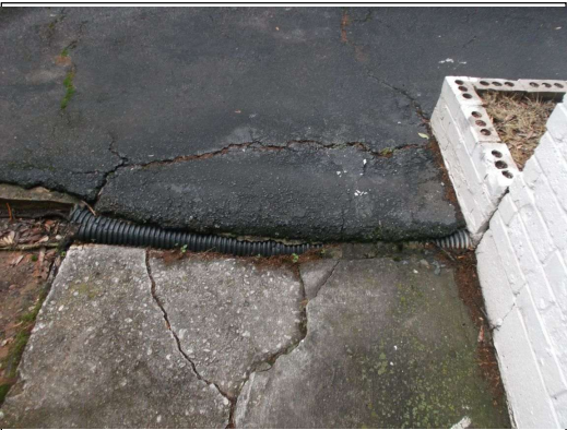
Walkway at the driveway broken trip hazards
