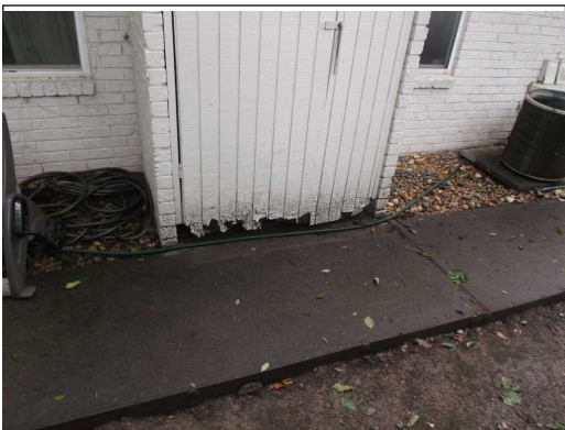
Doors rotted at the 2nd meter room
