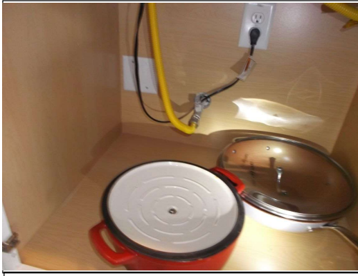
Gas pipe extends into the storage area
