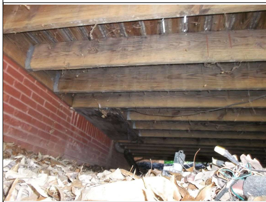
Deck bolted to brick and cantilever
