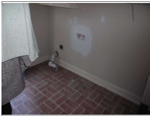
No washer drain pan
