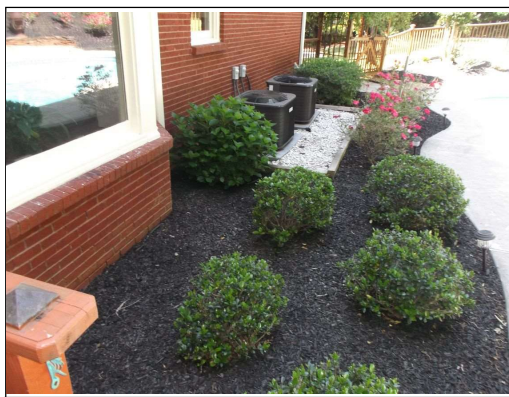
Ground slopes to the foundation
