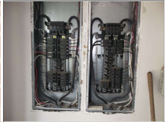
Openings at the bottom of the panels
