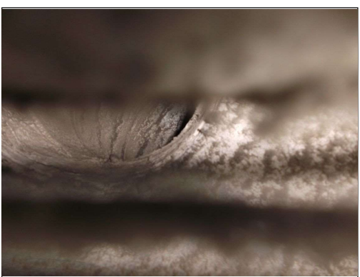
Air ducts rusty
