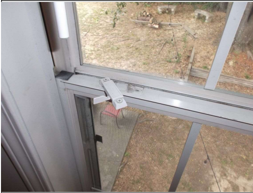
Detaching window lock
