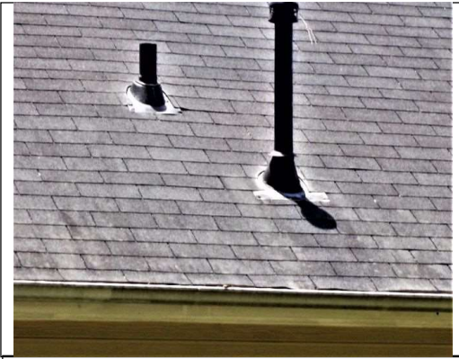
Pipe flashing on top shingles face nailed
