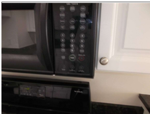
Microwave jell pad tarnished or soiled
