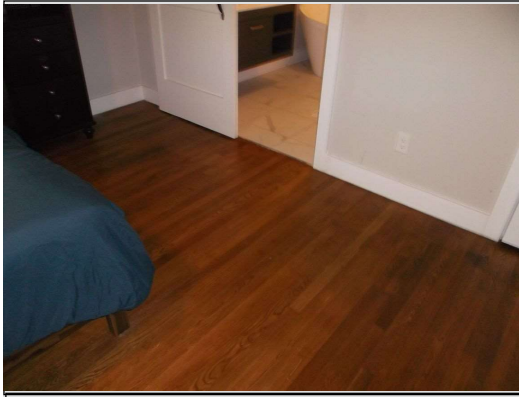
Master floor slopes to bath door
