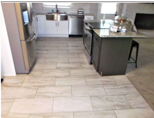
Floor sags and slopes to island
