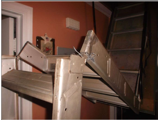
Attic ladder broken at the hinge (hazard)
