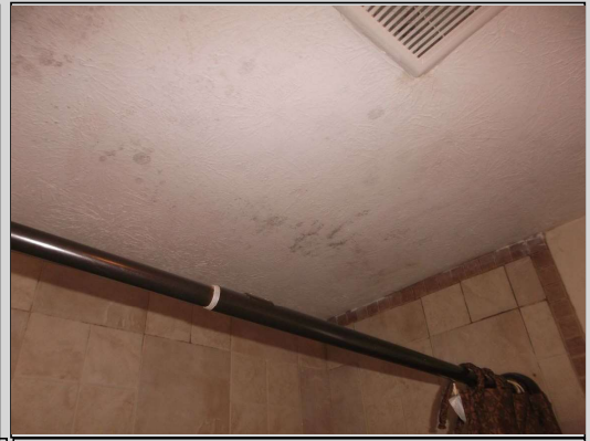
Bath ceiling has mold and sagging
