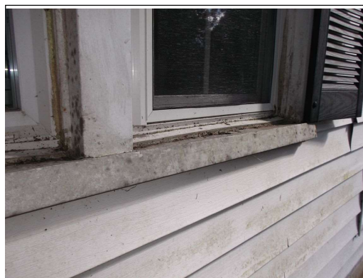
Cladding on seal slope to window
