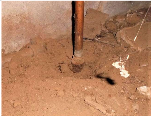
Main water pipe appears to be steel
