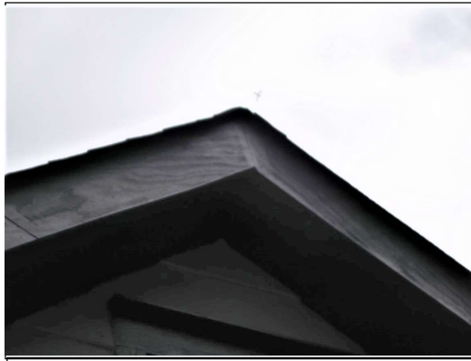
Fascia made of plywood/missing drip flashing
