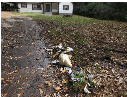
Water leak in the front yard
