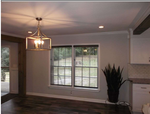
Ceiling sagging over window area
