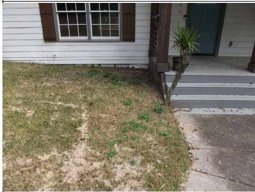
Soil slope to porch and foundation
