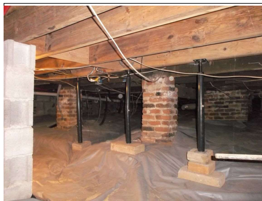
Jack posts placed under floor framing
