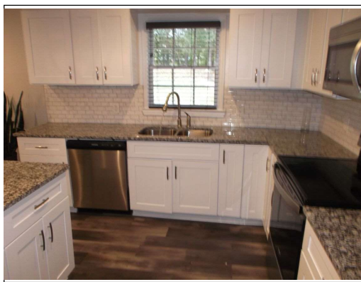
Counter and floor slopes to the left
