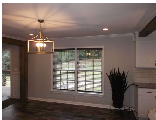
No air vents at exterior wall
