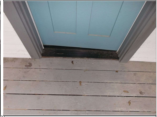
Front door threshold is not supported
