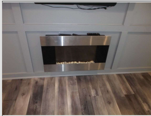
Verify fireplace operational
