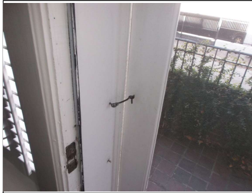
Hook not closing screen door fully
