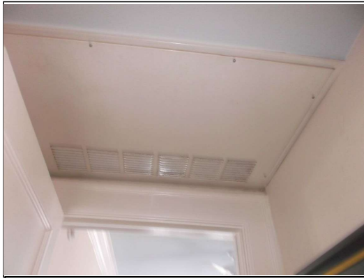
Furnace & filter covered with panel & screws
