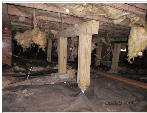
Many support Posts rest on blocks
