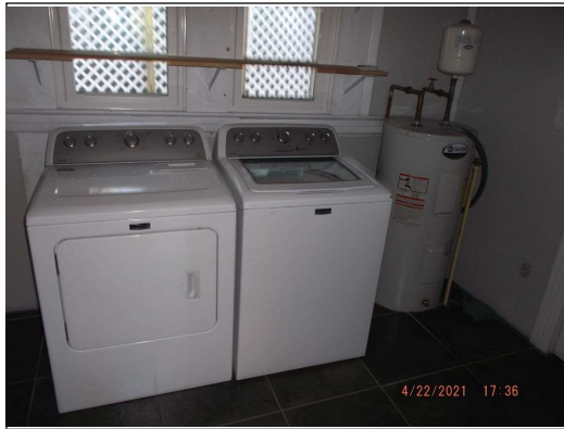
No washer drain pan
