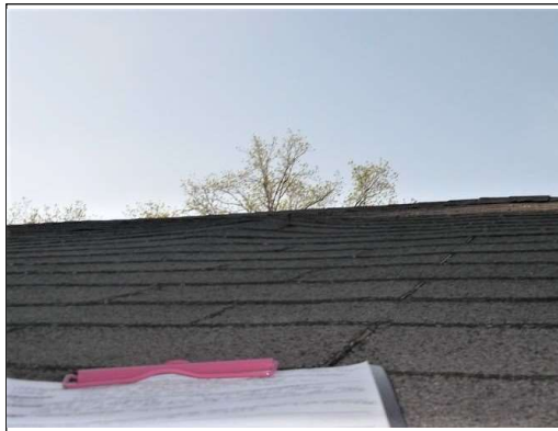
Hump and nail extracting at 2nd level room
