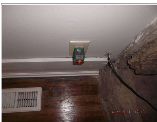
Outlet tested open ground at living room
