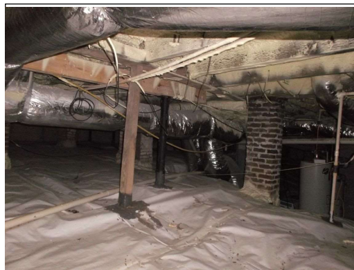
Floor covered with foam
