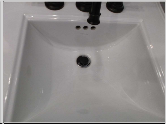
Finish peeling of drain outlet
