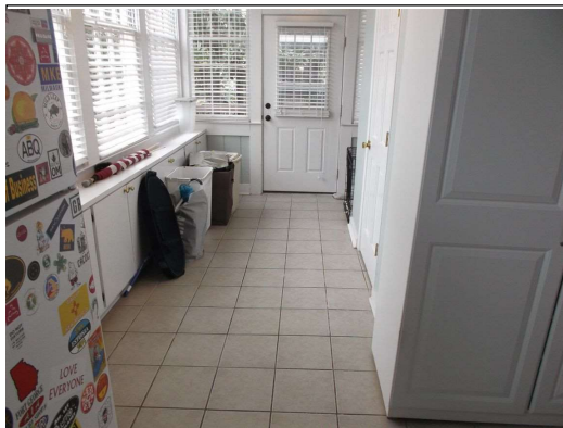
Laundry floor slopes to the left
