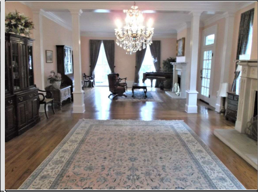
Floors settle and sagging
