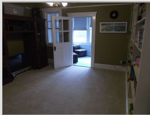
Floors major sloping and settling
