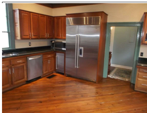
Base cabinet doors bump right of D/W
