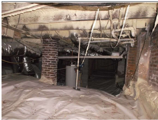
Foam cover floor framing
