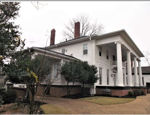
Building will need painting soon
