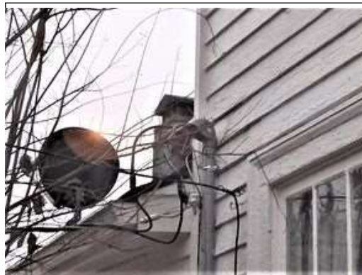
TV dish bolted to roof
