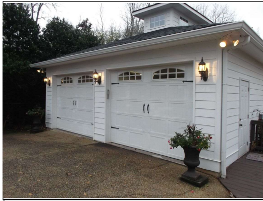
Doors need painting
