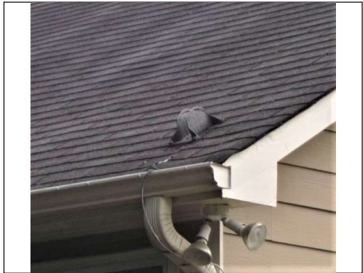
TV dish bracket bolted to the roof
