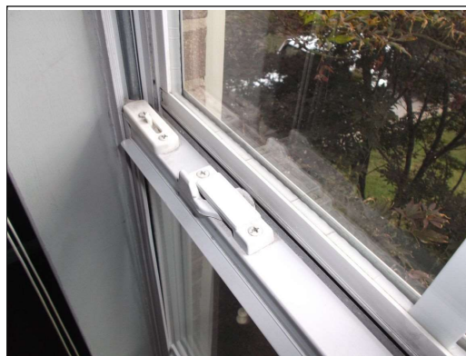
Master bed window lock not latching
