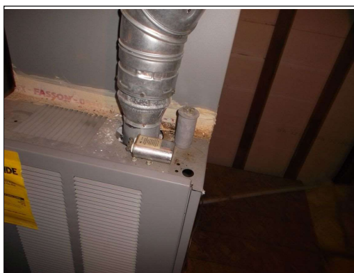
Furnace components have been replaced
