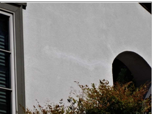
Cracks in stucco filled and painted
