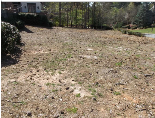
No ground cover soil erosion protection
