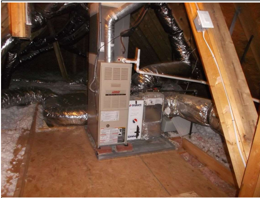
Attic furnace older model
