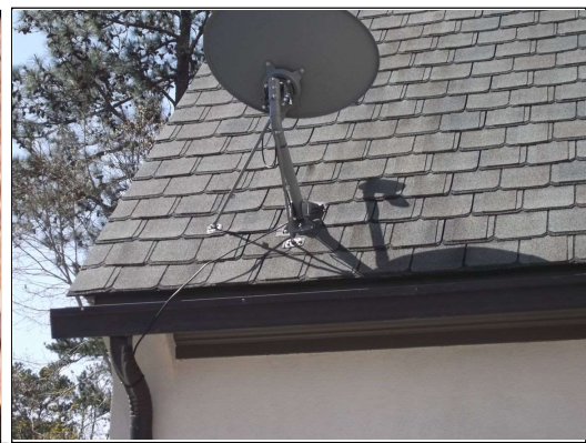
TV dish bolted to the roof at the rear of house
