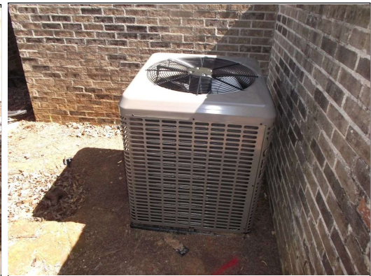
Poor clearance around at AC
