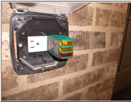
Basement patio outlet tested open ground
