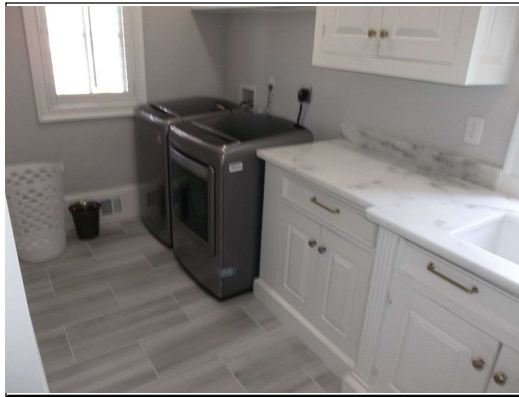
No washer drain pan installed
