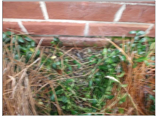
Soil contact brick & mortar can cause damage
