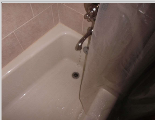
Tub stopper missing
