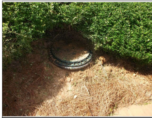
Verify if there is a septic tank at the rear yard
