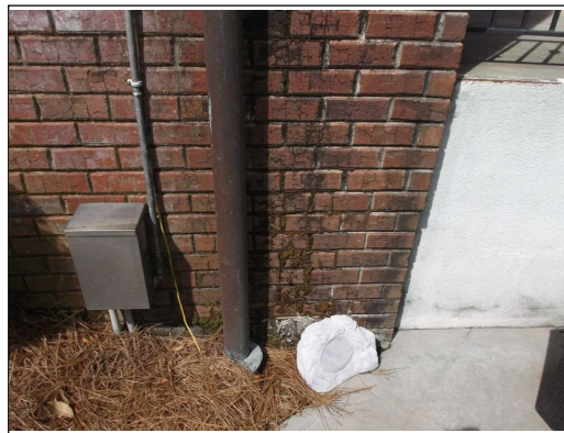
Algae on brick from leaking or overflow gutte
