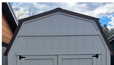
BARN STYLE ROOF
