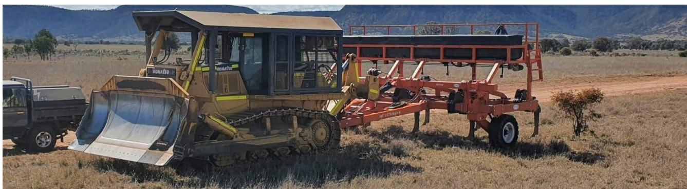
DOZER-DRAWN RIPPER RENOVATING PASTURE COUNTRY
