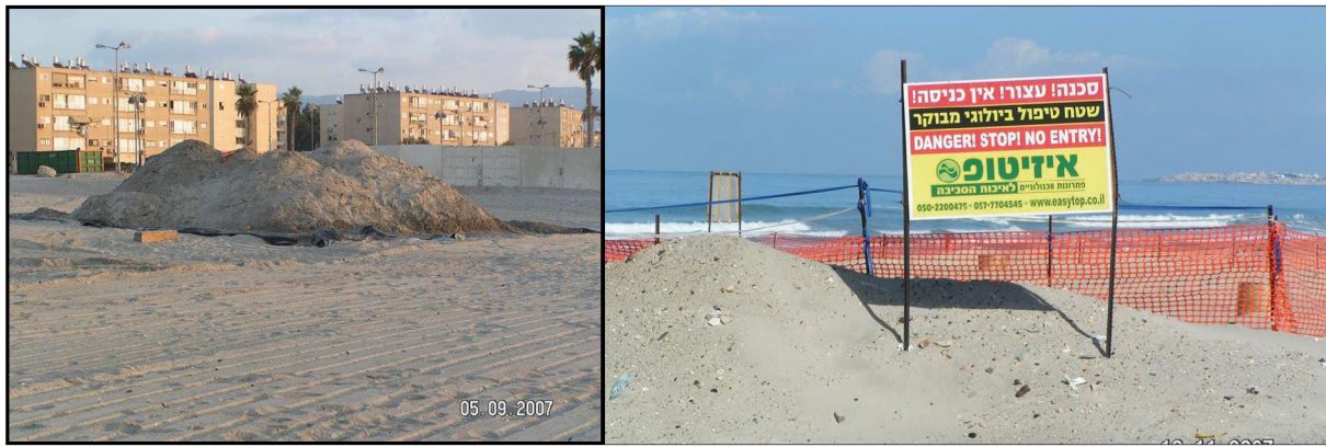
Figure 1. Initiation of the project on the Kiryat Haim beach. Note the polyethylene sheets underneath the contaminated sand piles.
