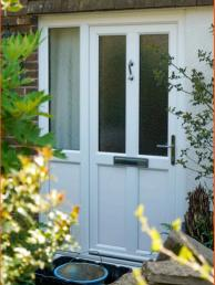
PVCu doors are made from a uPVC skin making up the exterior and interior of the door, with a Styrofoam core for good insulation whilst being light in weight. These doors can have a smooth finish in any colour or a natural look woodgrain finish (in a set range of colours).
