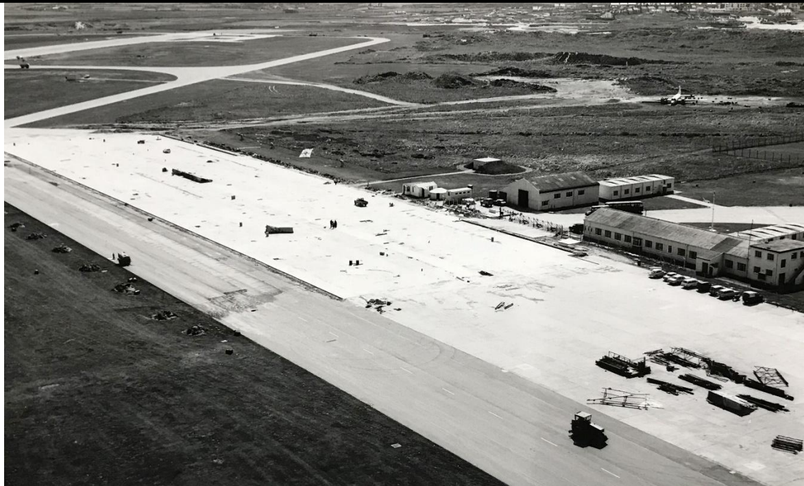
The STCAAME/MPC apron can be seen during the re-surfacing. The Varsity on the fire dump can be seen top right. [National Archives]
