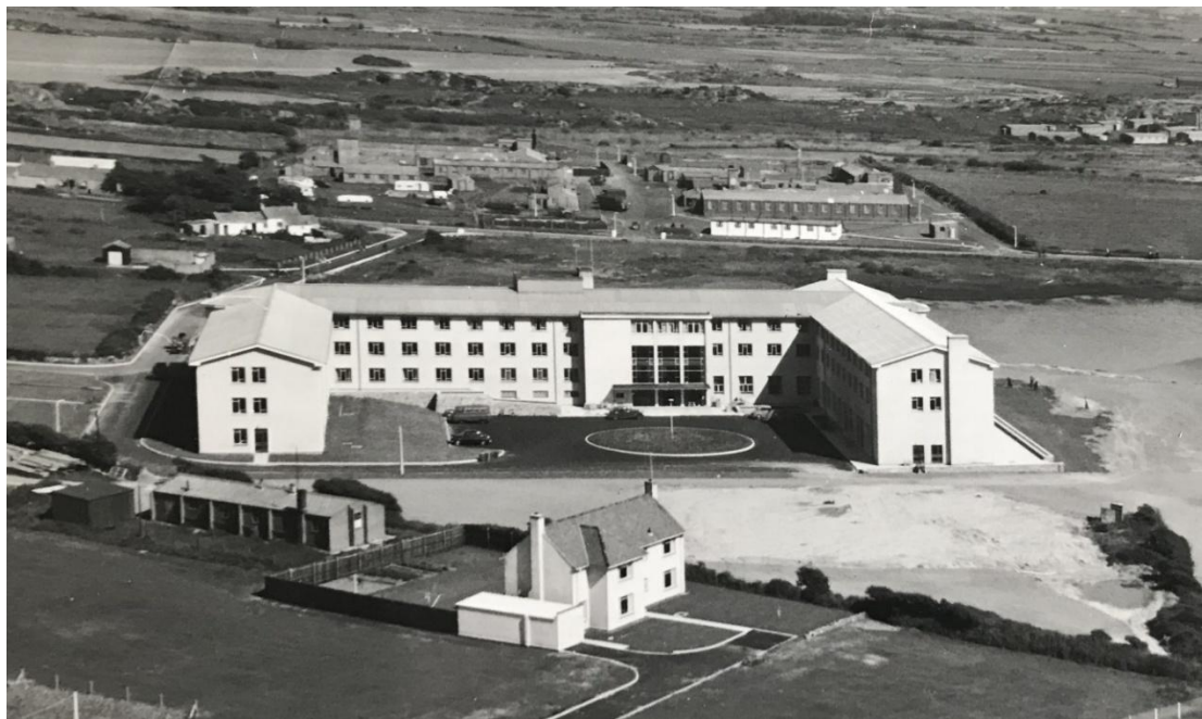
In this view Site 8 sleeping quarters long since demolished can be seen in the far right background.
