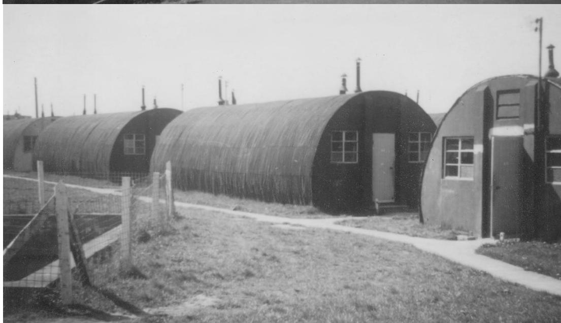
Although undated, these would appear to be one of the Sites by the Hotel Cymyran with Holyhead Mountain in the background in the top image and most probably sleeping quarters in the second image. [Dick Thomas collection]
