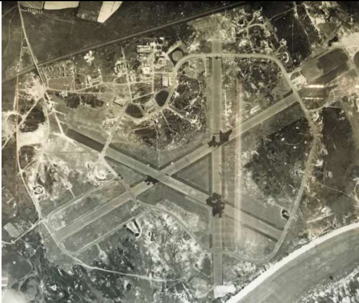
[Crown Copyright, Ministry of Defence]
