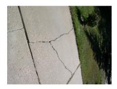
STEP 2 Clean the surface deep into the cracks and expansion joints. Using high pressure water blast the cracks are carefully cleaned. Actually done twice (first to just clean surface and cracks and then after grinding cracks etc.) We then us grinders and cutters to further clean the damage areas and prepare the surface for repair.
