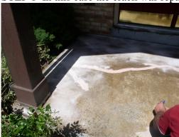
STEP 2. ShurBond 550 liquid was applied to the entire surface and while wet crystal sand was broadcast to rejection and the system allowed to cure and then the excess crystal is removed.
