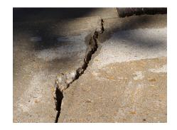
STEP 3 APPLICATION OF ShurBond 550 Epoxy Adhesive and ShurBond 100 Polymer Concrete to repair the surface. Rebuild expansion joints using high quality PolyUrethane Sealant.
