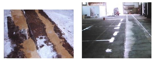
The photo shows a close up of the steel rail cover by ShurBond 500. The photo on the right shows one of the rail lines after smoothing with ShurBond 500. The area to the left shows concrete failure areas that have been repaired with ShurBond 500.
